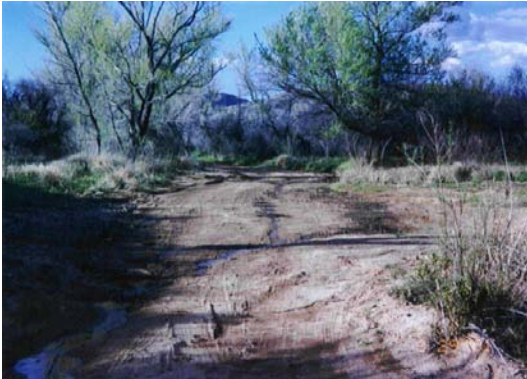
Photo JW-1-9 Direction: N Route: AF-12 Route in wash impacting riparian area in Badger Springs Wash .
