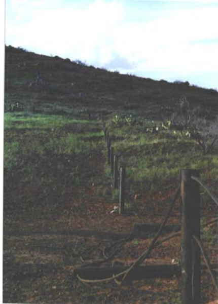
Photo: JA-1-2 Direction: NE Route: AF-14 Ineffective closure allowing ORV traffic into Agua Fria Canyon
