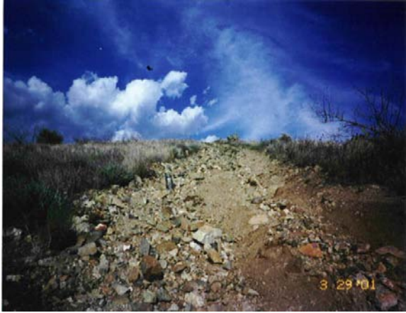
Photo: JA-1-5 Direction: E Route: AF-14 Severe erosion on steep route. ORV only
