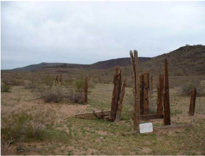
BT-1-64 old ranching structure in disrepair on route 19 Direction: W
