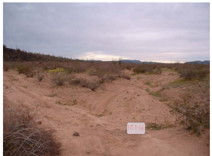
BT-1-66 worst erosion 24-36 inches on route 19 Direction: SE
