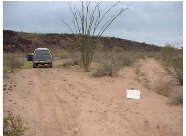
BT-1-62 Worst erosion and braided on route 19 Direction: NE
