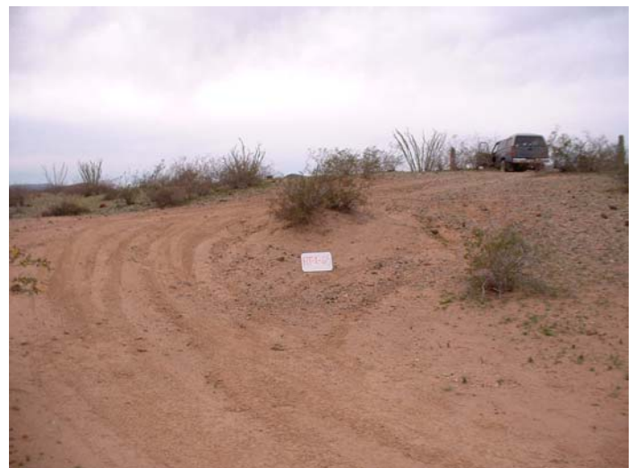
BT-1-65 worst erosion and braided route 19 Direction: NW
