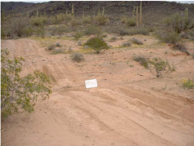
BT-1-60 worst erosion on route 17 Direction: E
