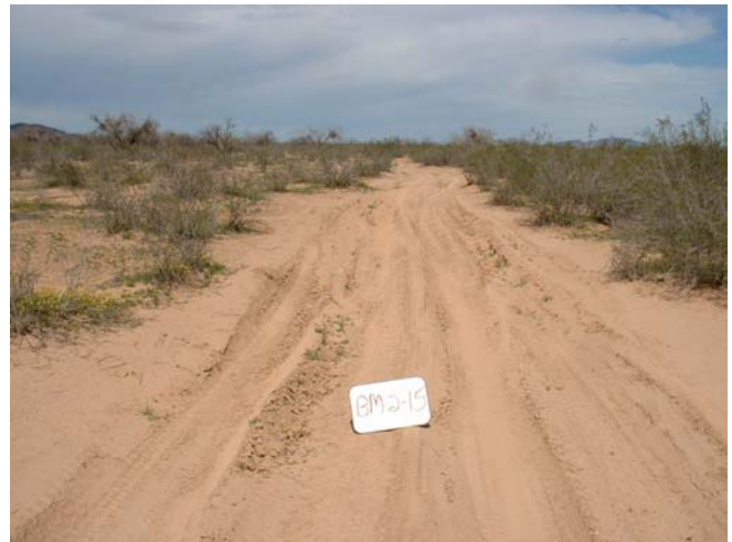
BM-2-15 Worst erosion, braided on route 12
