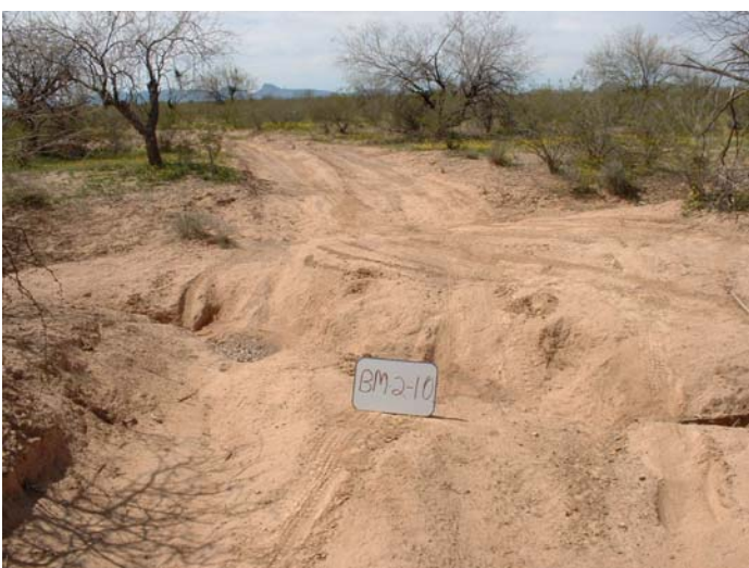
BM-2-10 Worst erosion on route 10 Direction: SW
