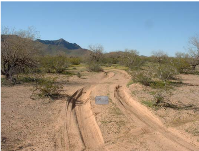
BM-2-32 Worst erosion on route 15 Direction: N
