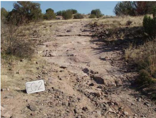
**EC-2** Erosion on route EC-A up to 15 inches.
