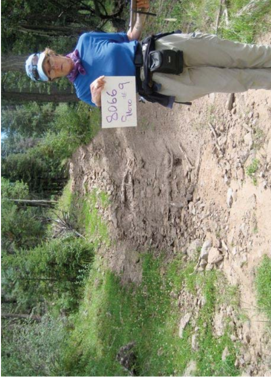
Photo 8066-9: Erosion on 8066 to north of Crackerjack Tank indicating unsustainable route location (GPS 671190, 3753887)
